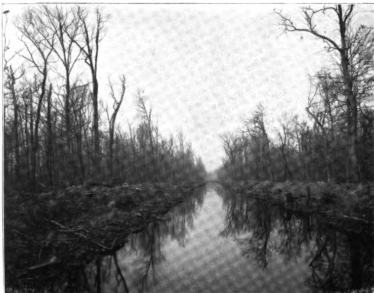
FINISHED DRAINAGE CANAL NEAR MOREHOUSE
